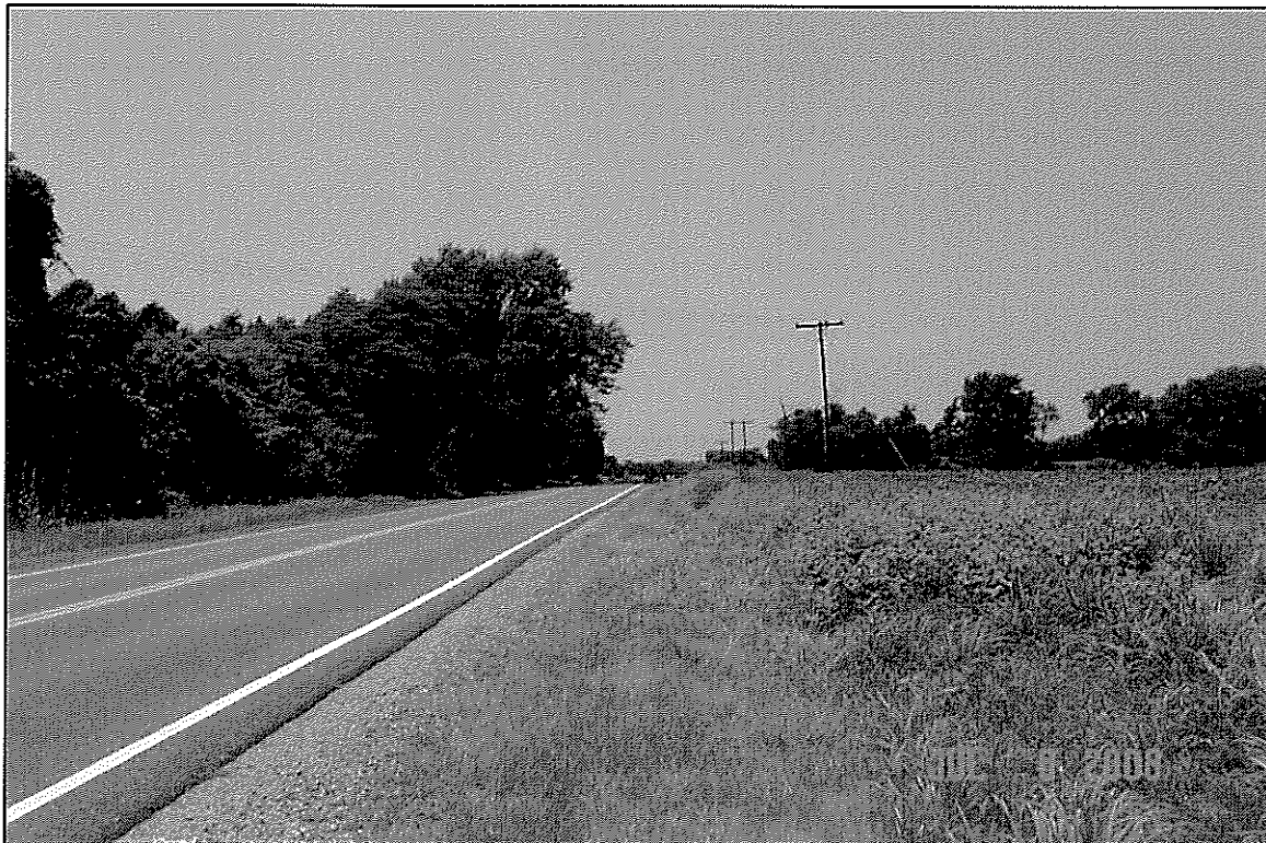
Looking to the north (Spotsylvania)
